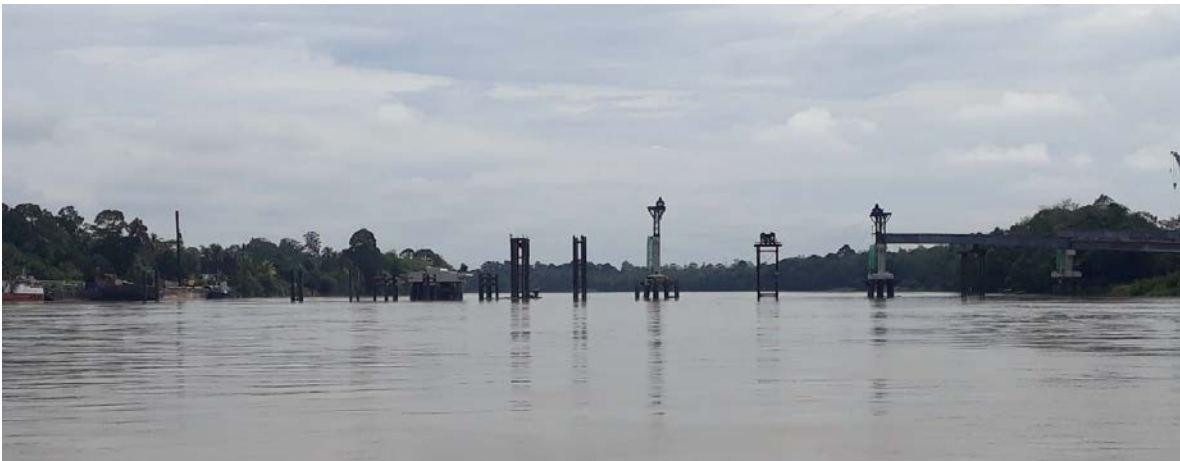
Figure 3 Bridge Construction at Samba
