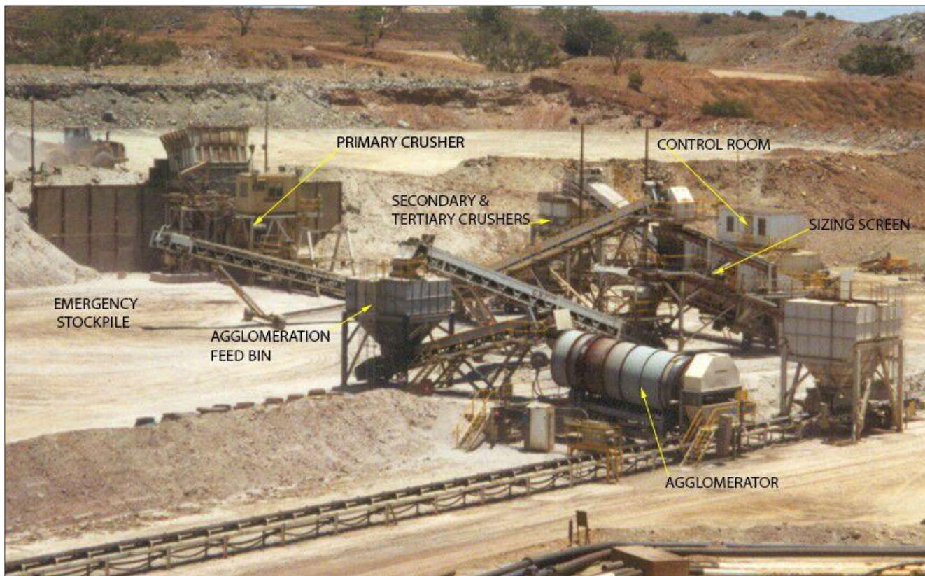
Figure 17-2 Typical small crushing and agglomeration plant
