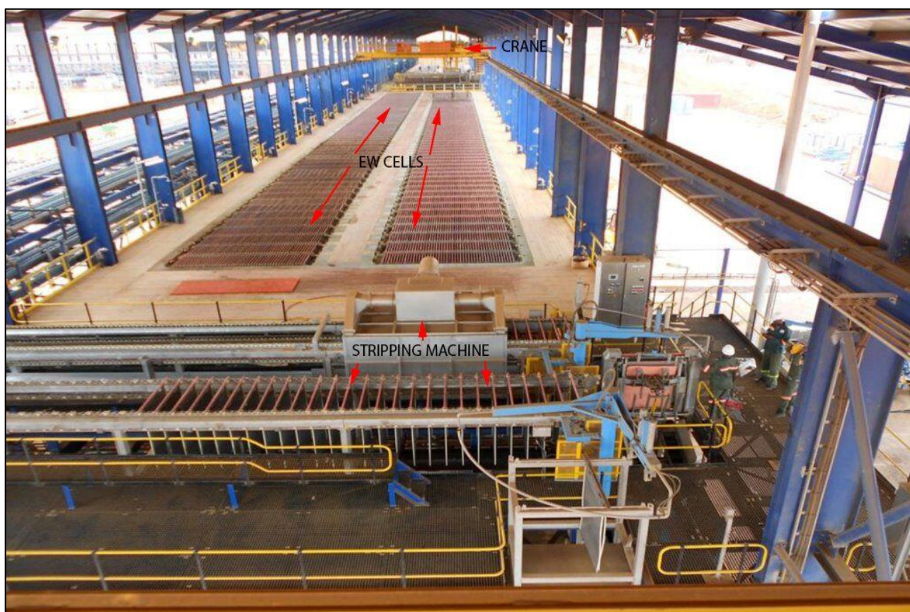
Figure 17-16 Internal View of Electrowinning Plant
