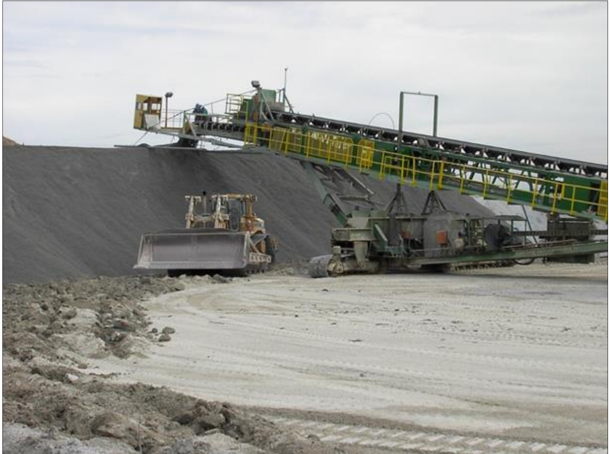
Figure 17-9 Stacker and Dozer Ripping the compacted surface
